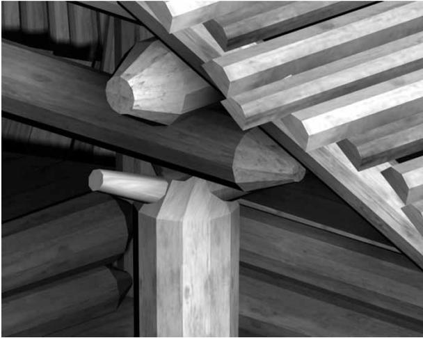
FIGURE 3. Post and beam construction, computer reconstruction.
